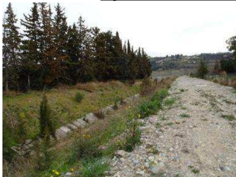
Figure 91 - Fossé en limite Nord © EGIS 2019
